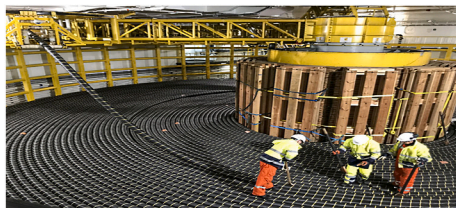
Fig. 4. Winding of a full cable length on a turntable in the factory.
